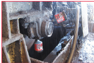
Bearing and seal lubrication on conveyor pulley bearing
